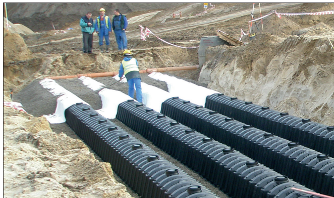
Figure 7 Installation of infiltration tunnels
